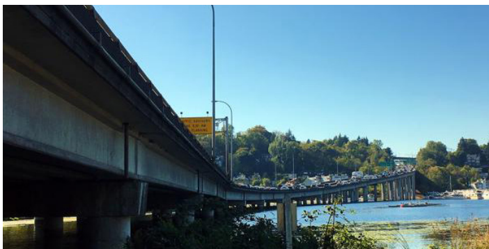
SR-520 bridge traffic in Seattle. Drain pipes visible at each column allow contaminated stormwater to flow directly from the roadway into Portage Bay, Union Bay, and Lake Washington. PHOTO: KATHY PETER
