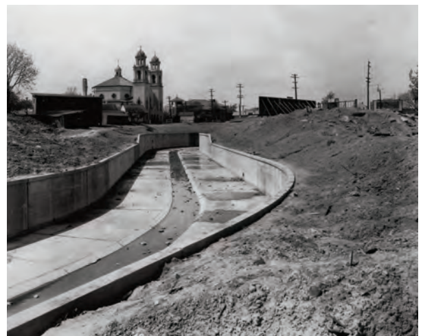
Trying to control flooding, the South Fork of Beargrass Creek was converted into an engineered channel, with a dry-weather channel running down its center.
