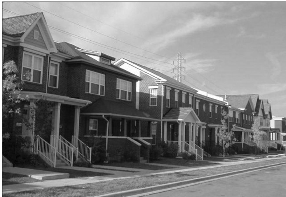
New housing in the Park DuValle neighborhood.
