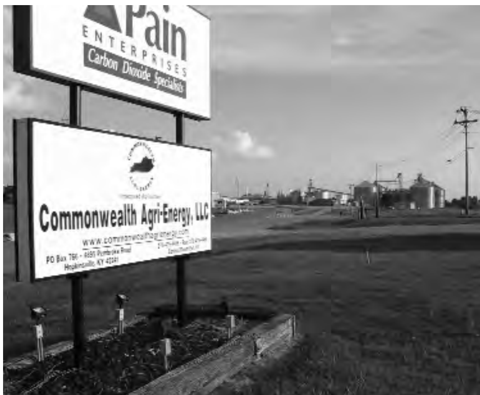
The Ethanol Plant in Hopkinsville, Kentucky.
