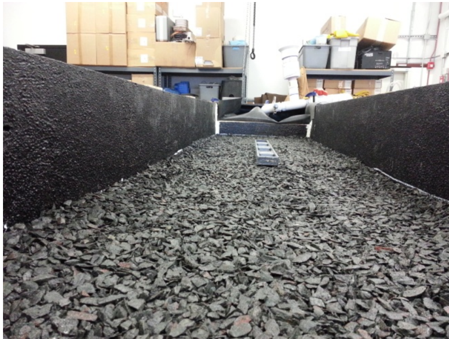
Figure 24: Compacted and leveled bedding layer
