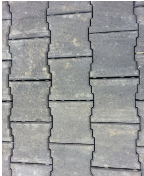
Figure 28: PaveDrain pavers in Louisville's CSO130 installation
