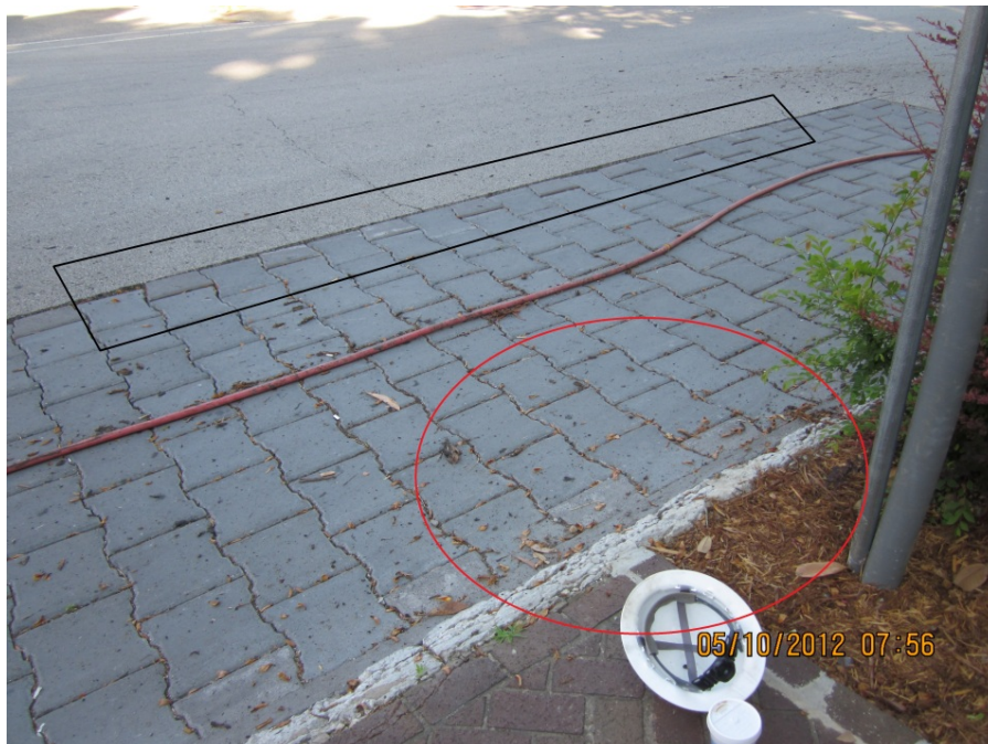
Figure 11: Segment A, 19 G, second maintenance
