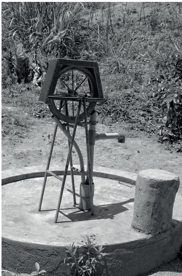
Figure 1. Rope and washer pump, Rumph District
