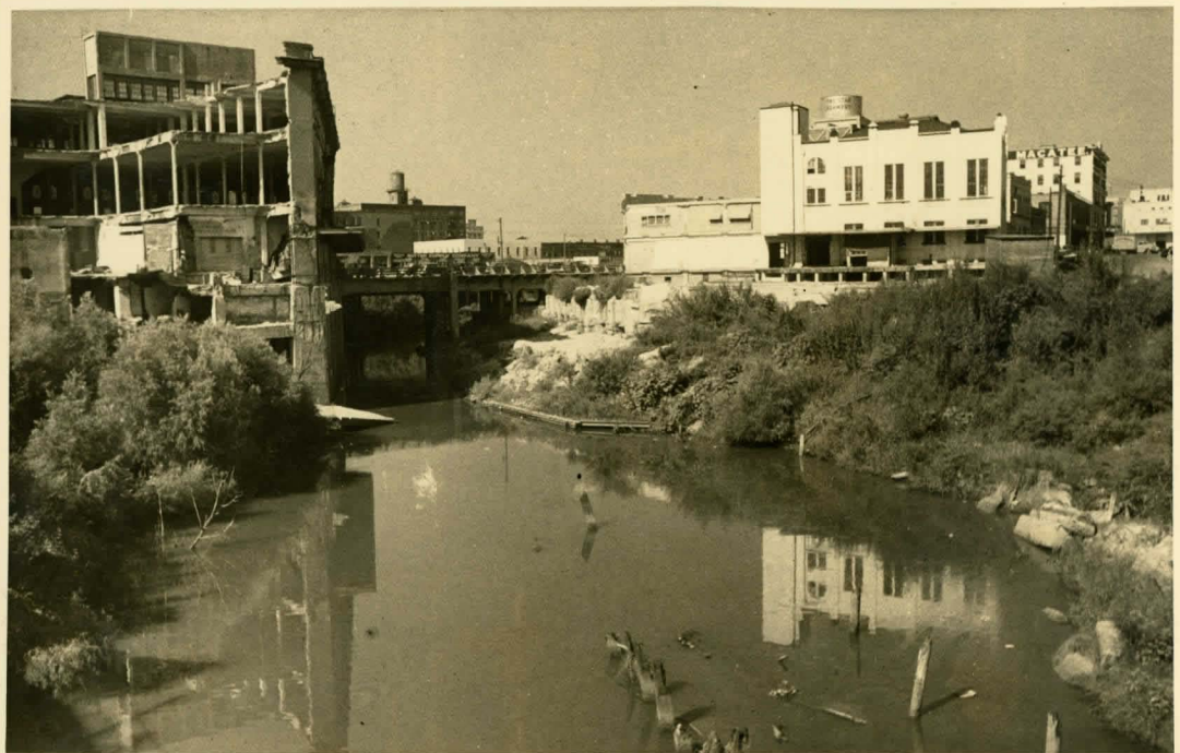
Fig. 4. Franklin Ave. Bridge; note the restricted channel and the buildings destroyed by the 1935 flood, view looking upstream.
