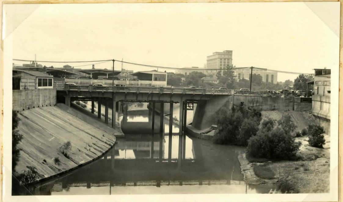
Fig. 6. The restricted channel at the Preston Avenue Bridge, looking upstream toward Farmer's Market.
