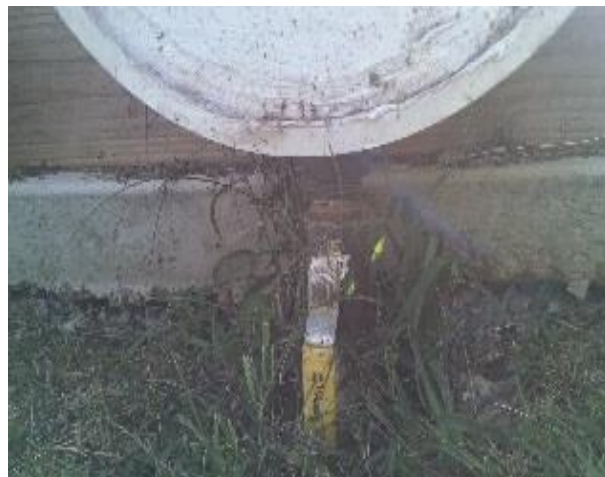
Figure 3.6 a Trough out Flow Valve
