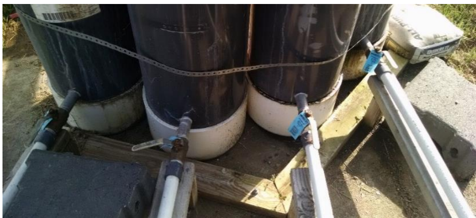
Figure 3.5 Outflow Control from Filters
