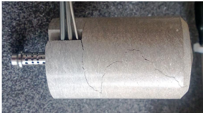
Figure 77 - Cracked nozzle insulation due to expansion at elevated temperature
