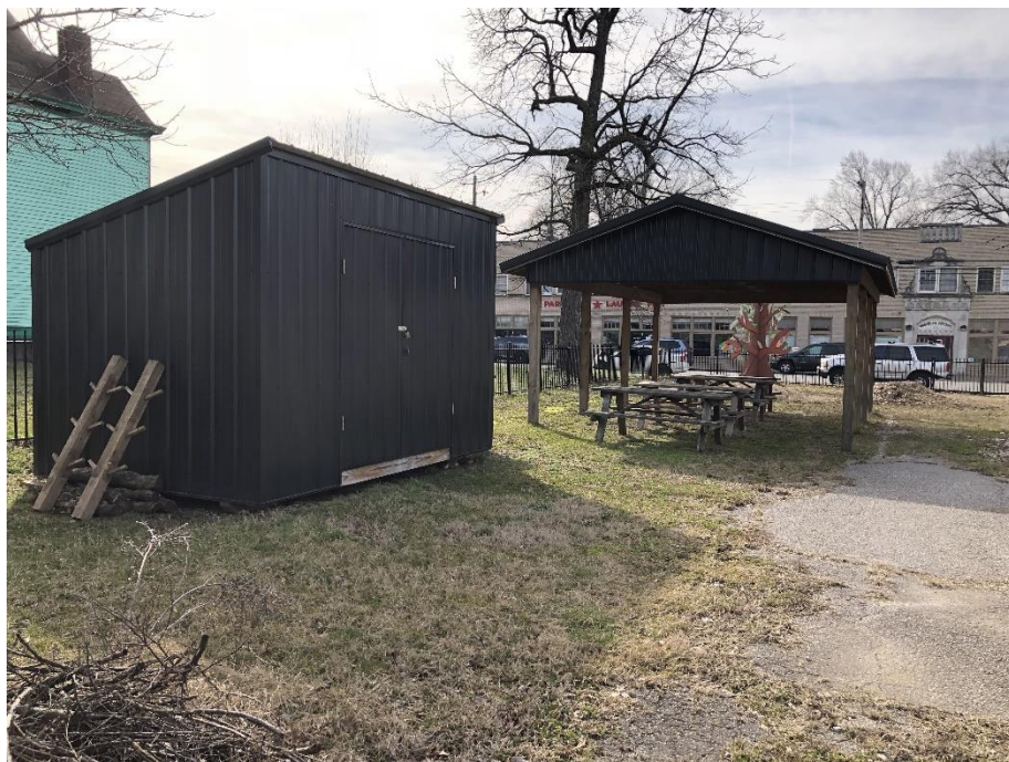
Figure 4: Parkland Community Garden's tool shed and covered shelter. February 2019.
