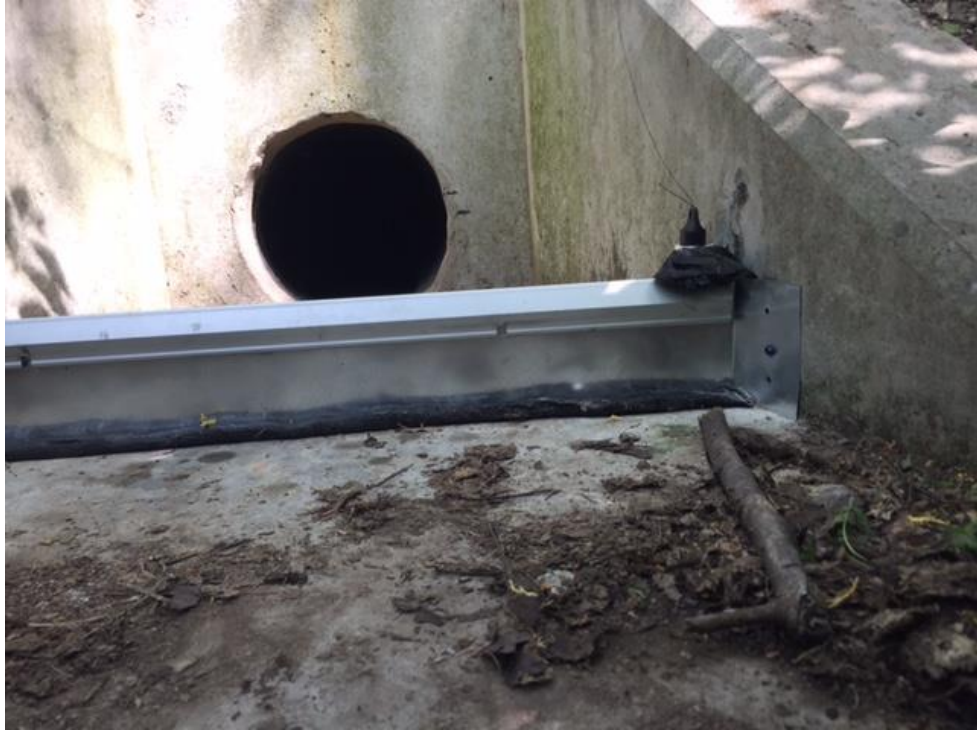
Figure 20. The weir installed in front of the headwall in UGF-1.
