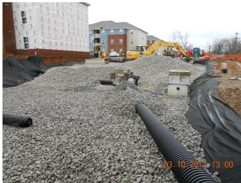
Figure 10. A non-woven geotextile is being placed on the bottom and the walls of the basin.
