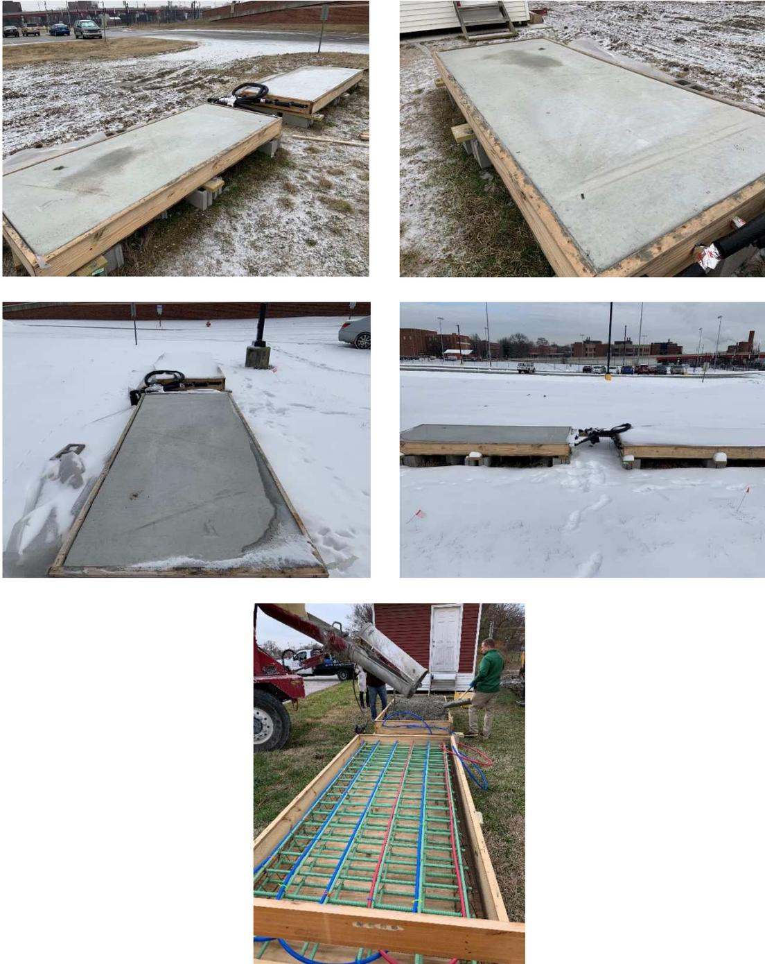
*Figure 1-1 Bridge deck de-icing project, using geothermal energy*
