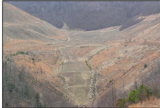
Figure 1. Valley fill (a) prior to watershed retrofit (2007), (b) stream channel construction utilizing natural channel design (NCD) techniques (2008), and (c) implementation of forestry reclamation approach (FRA) principles. (Images are courtesy of University of Kentucky)
