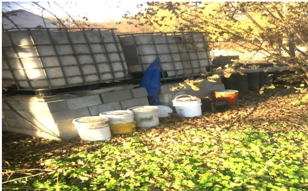
Figure 7. Rainwater harvesting (1200 gallons in both tanks) at Lots of Food Garden, in the Portland Neighborhood, West Louisville. November 2021. (Photo by Sait Sarr)
